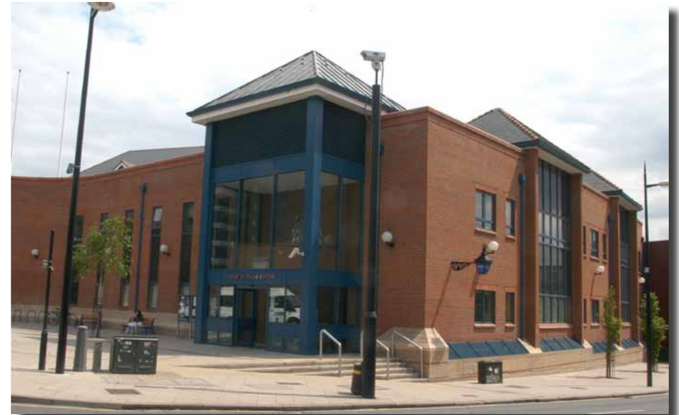
Bromley Police Station - a modern multi-purpose building
