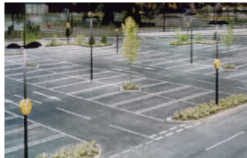
▲ Good lighting of a car park with no shadows, light pollution or glare.
