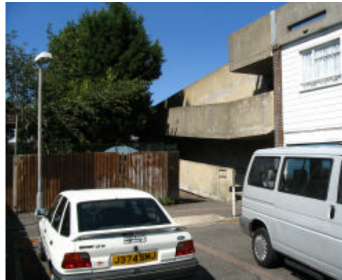
▲ Obscured access routes, such as this walkway, can lead to under-used, isolated and unsafe environments
