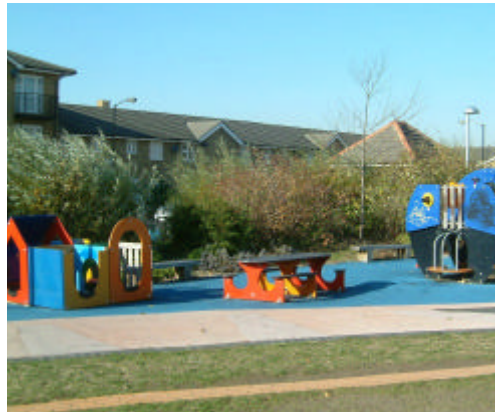
▲ Children's play areas that are not able to be observed are vulnerable to graffiti and vandalism
