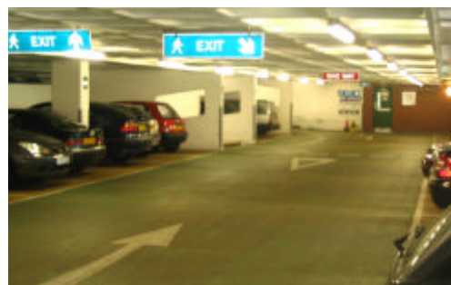
▲ Good lighting and clear signage in Gibson Road multi-storey car park maximises natural surveillance and avoids shadowed areas
