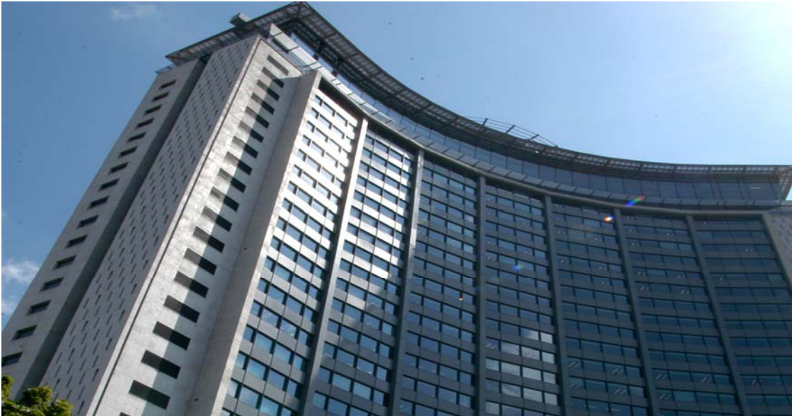
Empress State Building Houses a range of operational and non-operational functions
